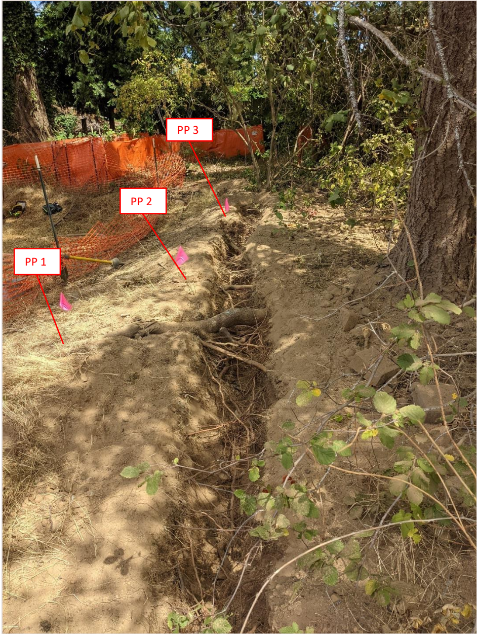
Figure 2. Excavated trench (photo looking north) showing Photopoints (PP) 1, 2, and 3.
